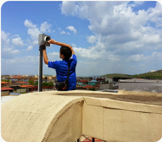
Exterior camera installation
