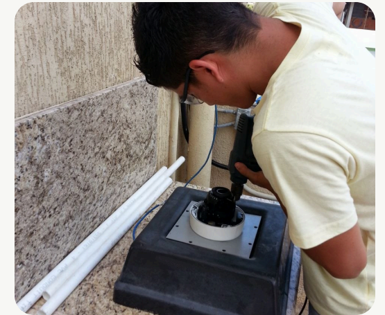
Cabling pathway and conduit detail
